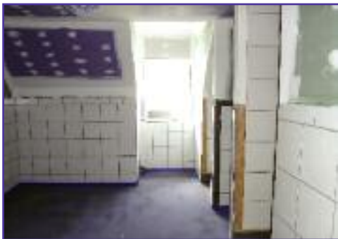
The bathroom renovation in progress
